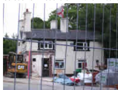
Work underway at the Lord Nelson
