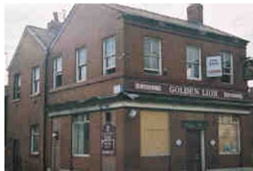
Work underway at the former Golden Lion
